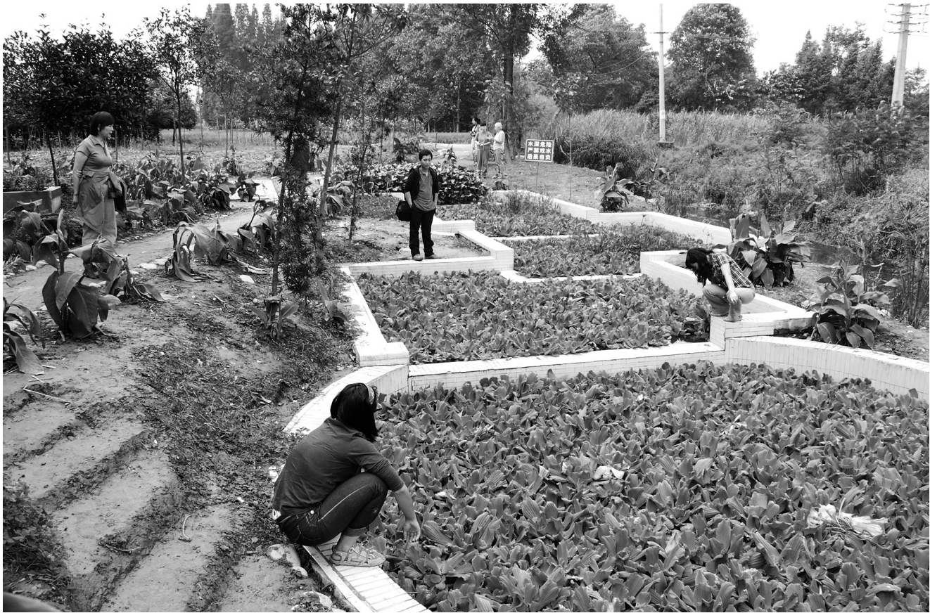
Fig. 6. Wetland constructed by the Chengdu Urban Rivers Associations to purify greywater proximate to an elementary school in Ping Yi County, Sichuan, China. (Photo © Betsy Damon) Inspired by Betsy Damon's Living Water Garden , 2010; < www.keepersofthewaters.org >.
